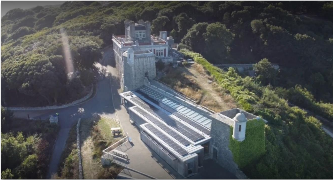
Figure 5: Aerial view of installed solar panels
