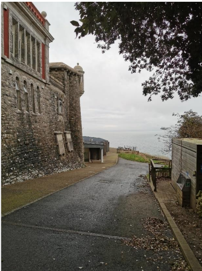
Figure 1: Durlston Castle before solar panels installed.
