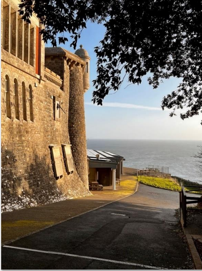
Figure 2: Durlston Castle showing solar panels installed.
